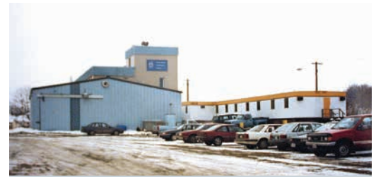
Old Metallurgical Technology Centre – Falconbridge, Ontario
